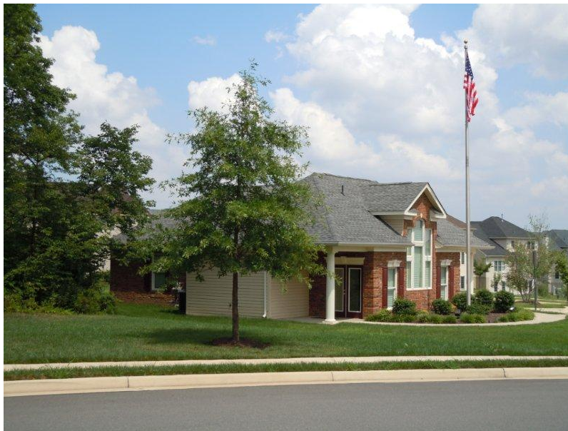
Exhibit 5-2: Photo of Flagpole at Civic Center (Height: 35.2’)
